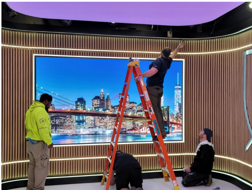
Figure 1 - Crew installing a digiTHIN HD Screen with ZEUS™
